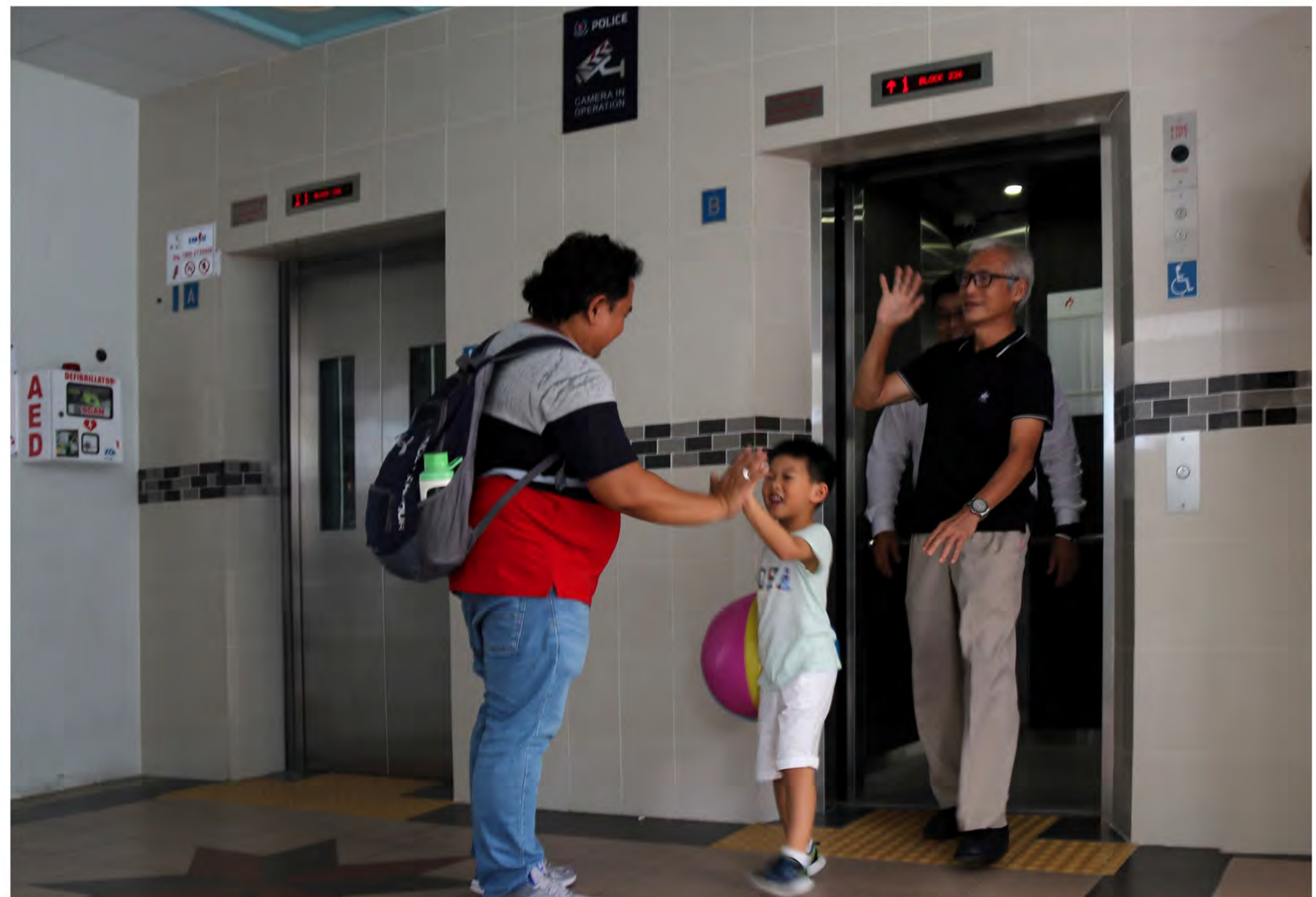
Upgraded lifts under the Lift Enhancement Programme at Blks 371, 372, 374 Bukit Batok St 31 and Blks 513, 514, 536, 537, 539, 540, 541 Bukit Batok St 52
