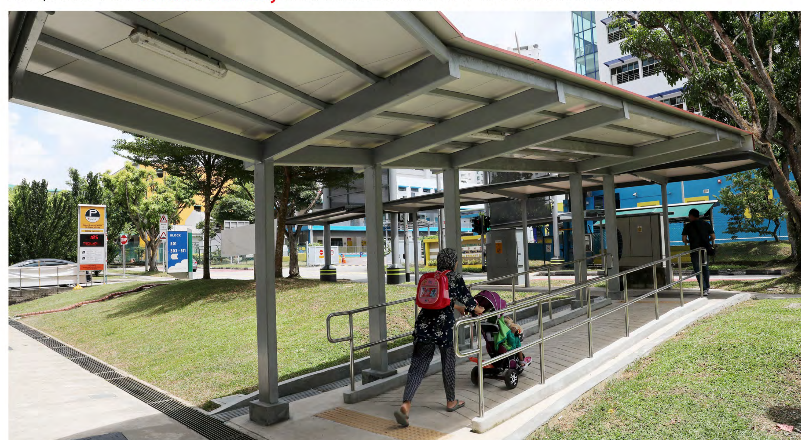
Sheltered linkway for residents and students at Blk 510 Bukit Batok St 52
