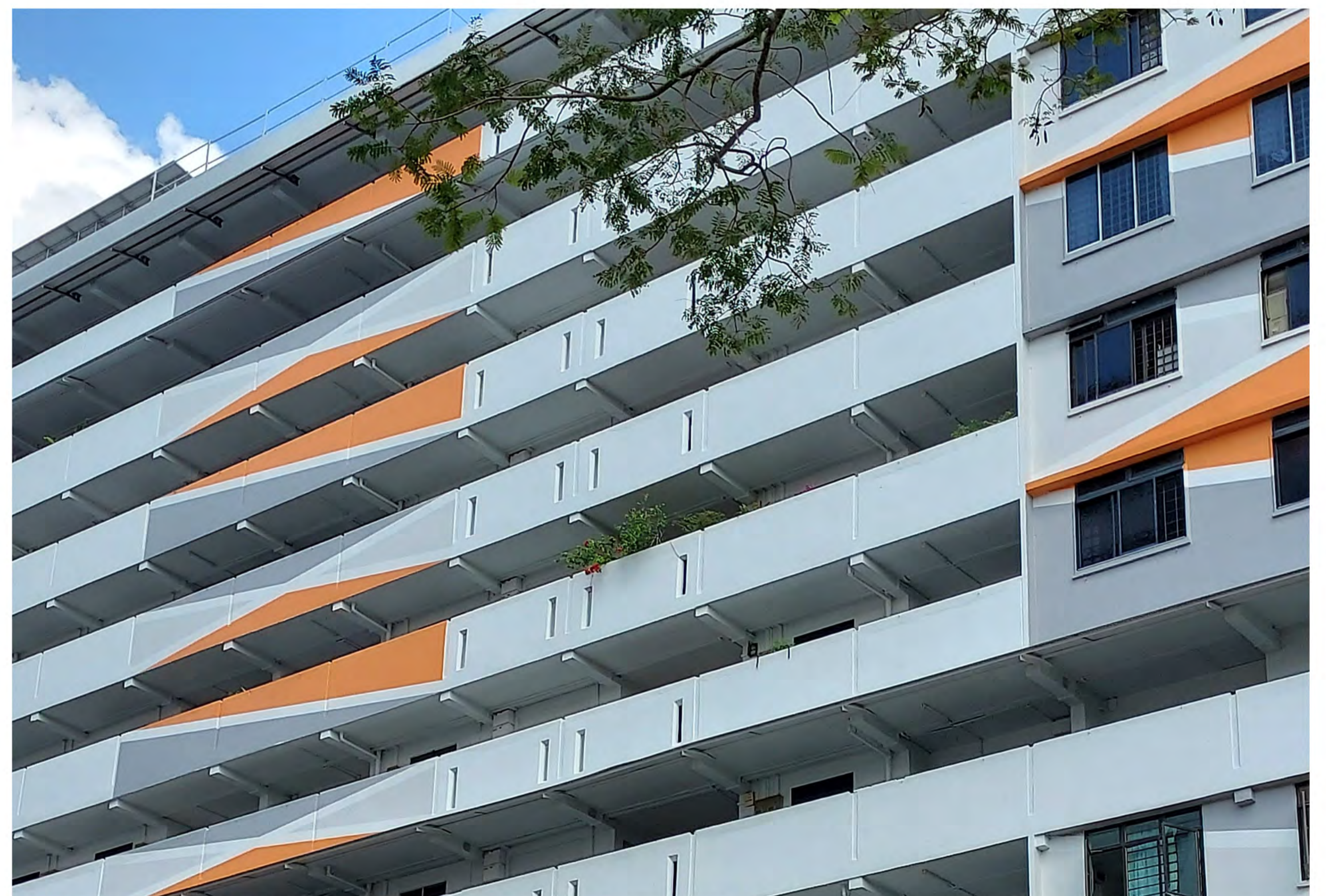
A new coat of paint for Blks 501, 503 to 511 Bukit Batok St 52
