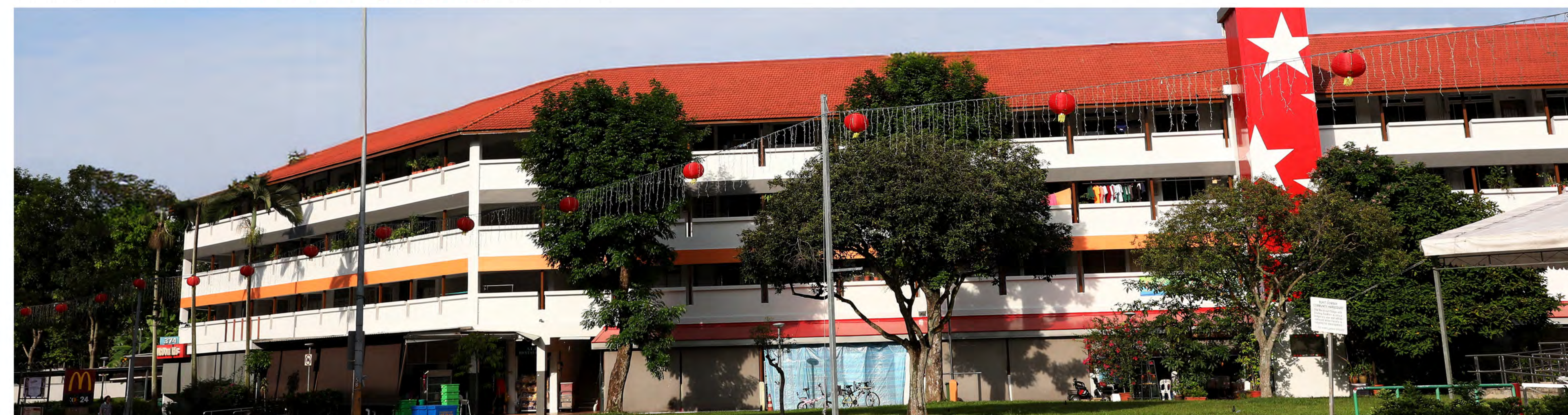
Blks 371, 372, 374, and 375 Bukit Batok St 31 will be upgraded with improved amenities under the Neighbourhood Renewal Programme (NRP)
