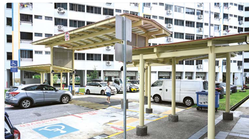
Linkway from Block 111 to 112 Teck Whye Lane
