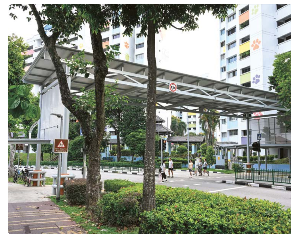
Linkway with barrier-free access ramp from Block 4 to 145 Teck Whye Avenue
