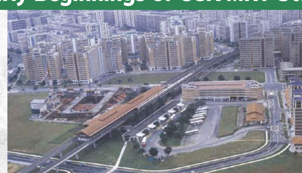
Aerial view of Choa Chu Kang MRT Station, Choa Chu Kang Bus Interchange and the public housing at Choa Chu Kang Town in 1996 Credit: All rights reserved, National Library Board
