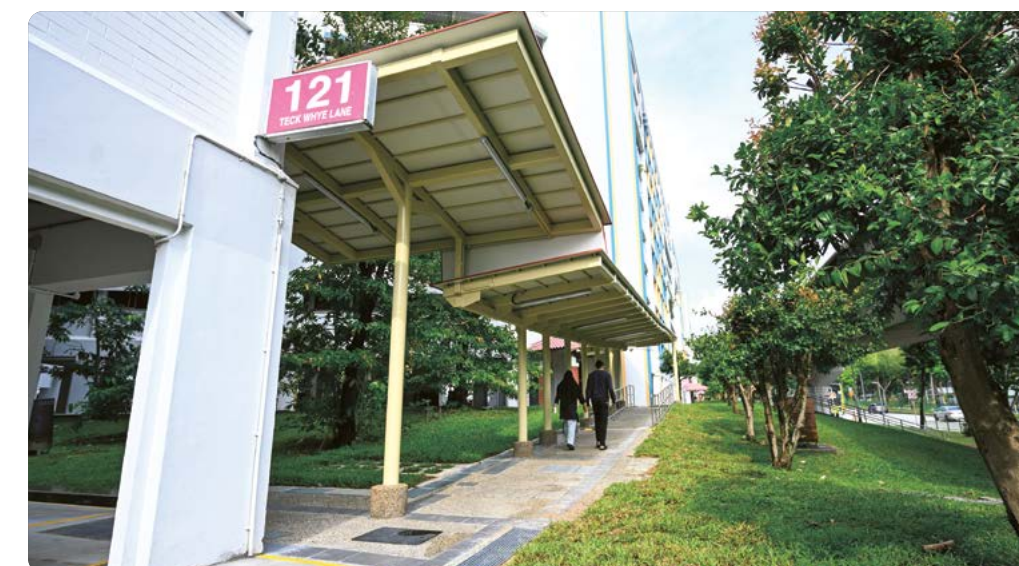
Linkway from Block 113 to 121 Teck Whye Lane
