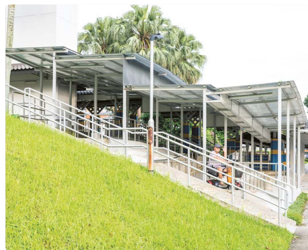
Linkway and ramp from Block 8 Teck Whye Avenue to bus stop
