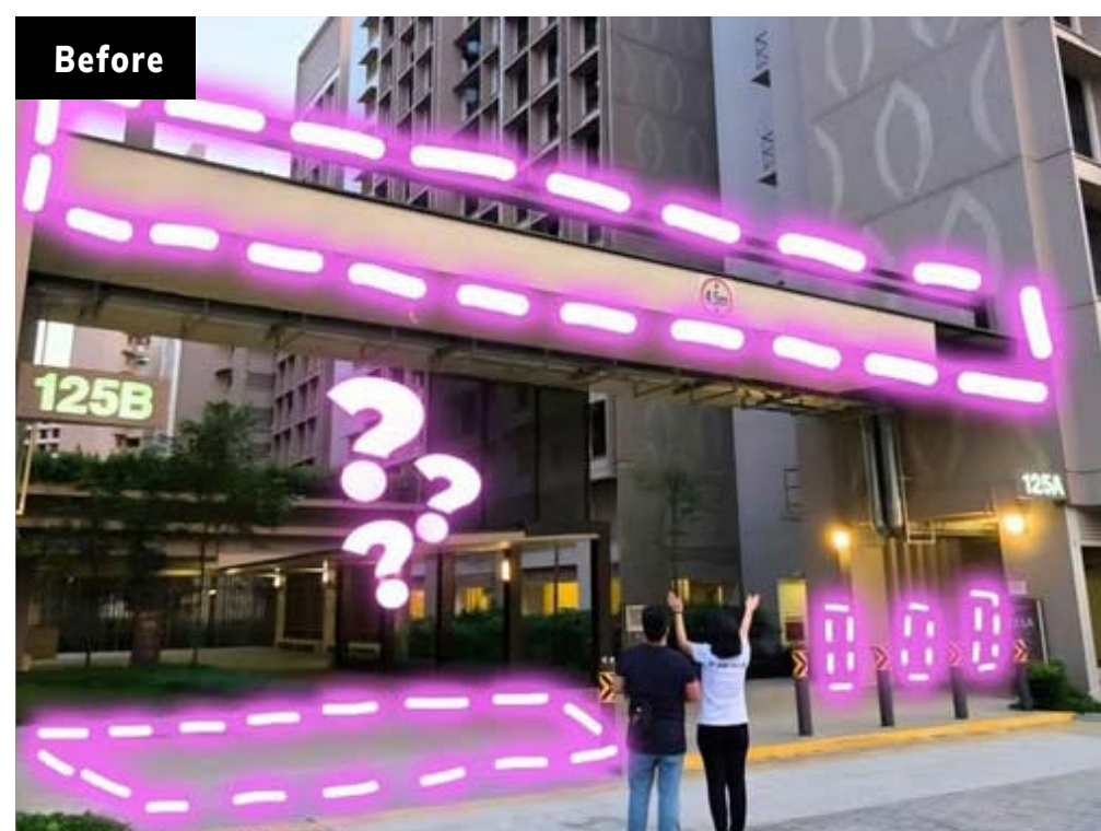
The drop-off porch at Blocks 125A and 125B Tengah Drive before the improvement
