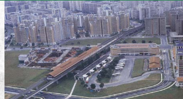
Aerial view of Choa Chu Kang MRT Station, Choa Chu Kang Bus Interchange and the public housing at Choa Chu Kang Town in 1996
